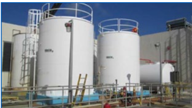
Double-walled Vertical Steel ASTs
