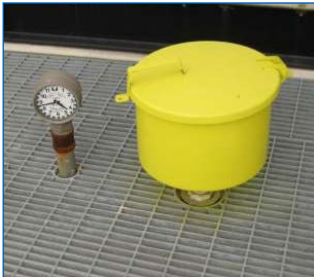
Clock Gauge Liquid Level Overfill Method
