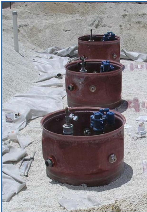
Pump Sump Installation
