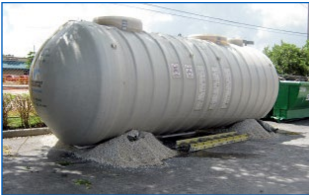
DW-Fiberglass UST Prior to Install
