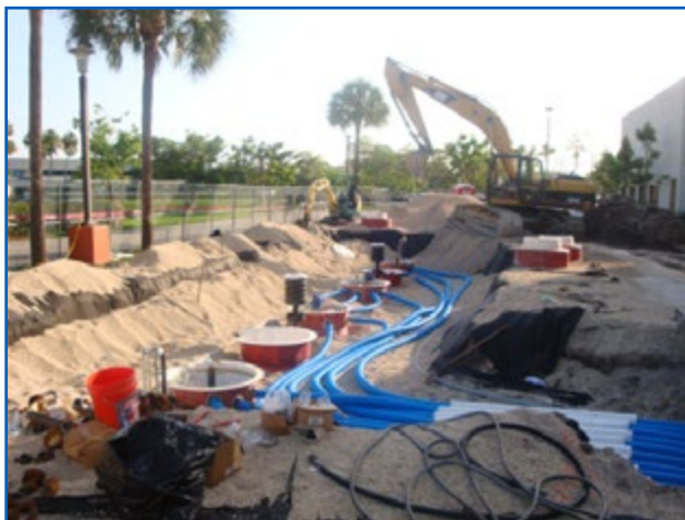
Double-walled Flexible Piping Layout
