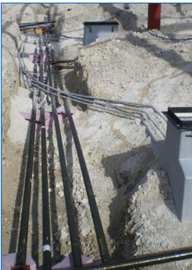
UST System Piping/Dispenser Liner Installation
