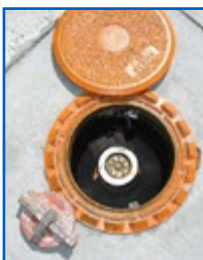
Stage I Vapor Recovery Color-coded Sump
