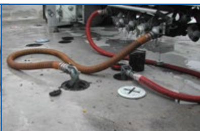
Fuel Delivery with Stage I Engaged
