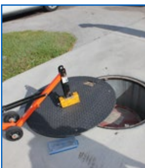
Pump/Piping Sump Manway Cover
