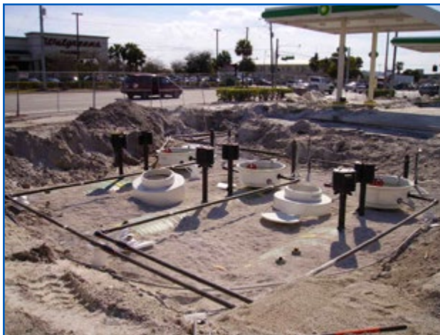
Double-walled Fiberglass Piping Layout
