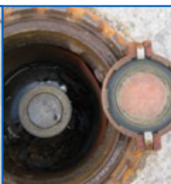
Stage I Vapor Recovery Color-coded Sump
