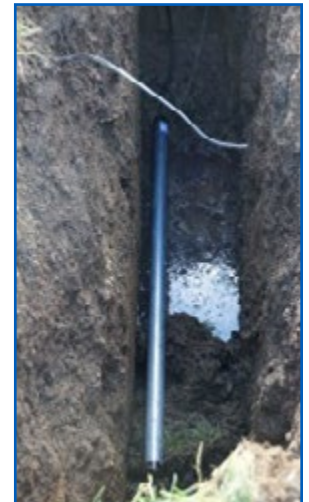
Sacrificial Anode Install
